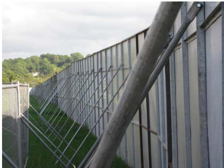
Fig. 10-4 - Solid temporary fence panels showing diagonal bracing. This is a pedestrian barrier used to channel queue lanes – perfect when no sideways pressure is anticipated. Photo courtesy of The Event Safety Shop, LTD.
